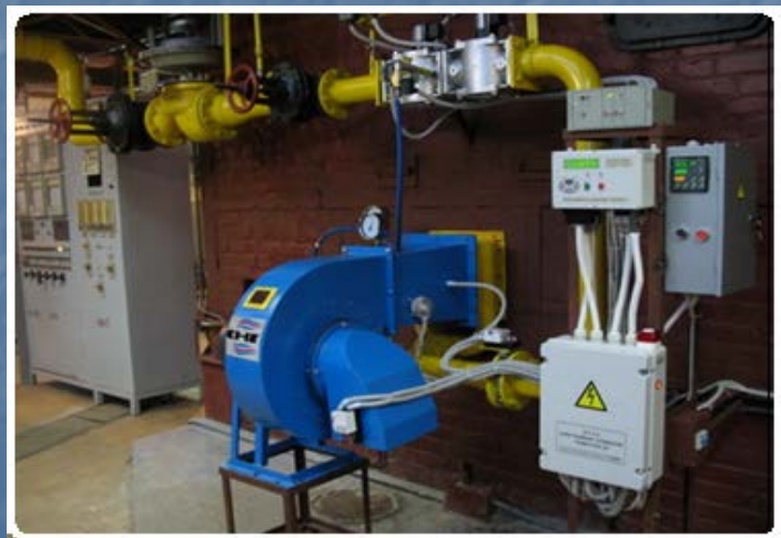
Burner device of stabilizer type to the boiler PTVM-50
