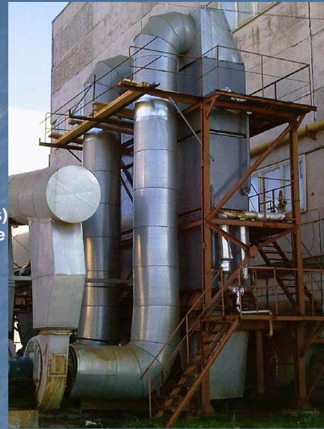
HEAT-RECOVERY SYSTEM FOR GLASS FURNACE
